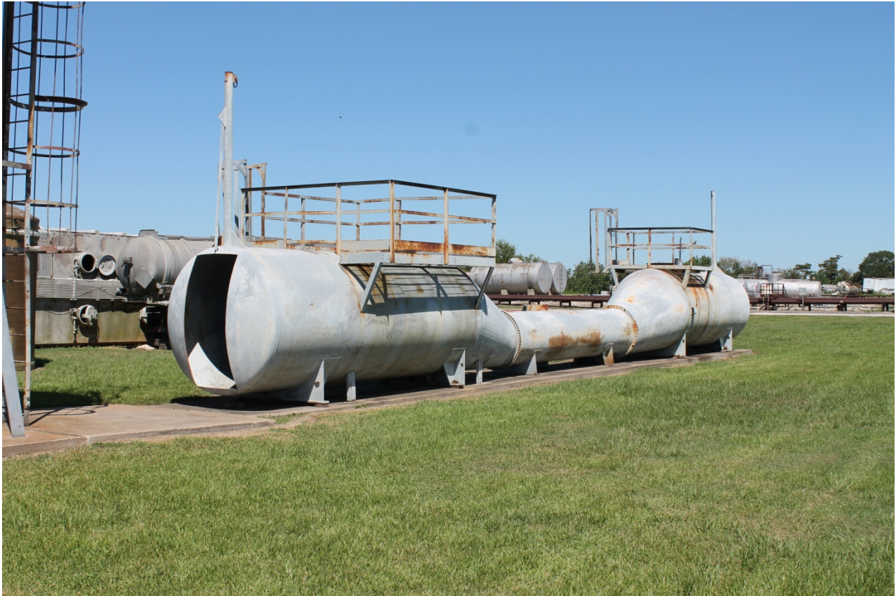
The confined space rescue vessel evolution
