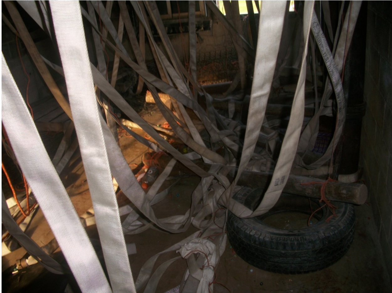
The second-floor obstacles
