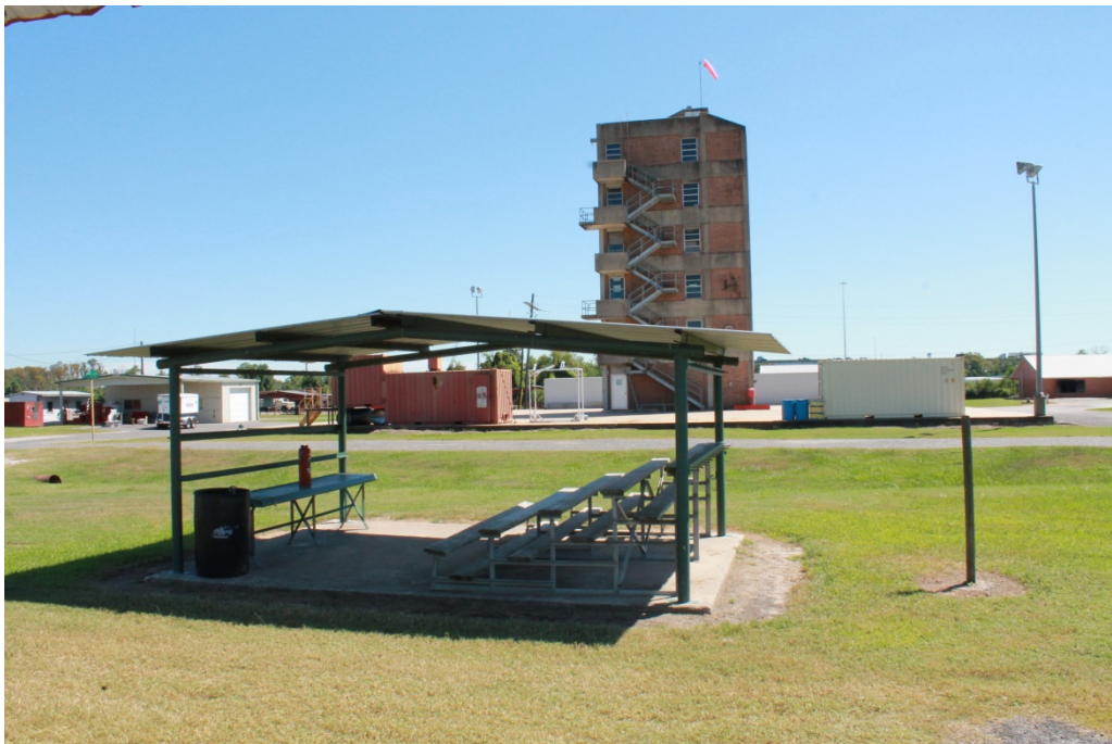
Staging and rehab for the smokehouse
